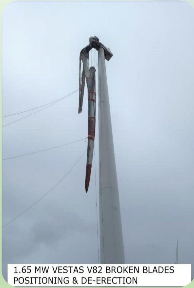
POSITIONING & DE-ERECTION 1.65 MW VESTAS V82 BROKEN BLADES
